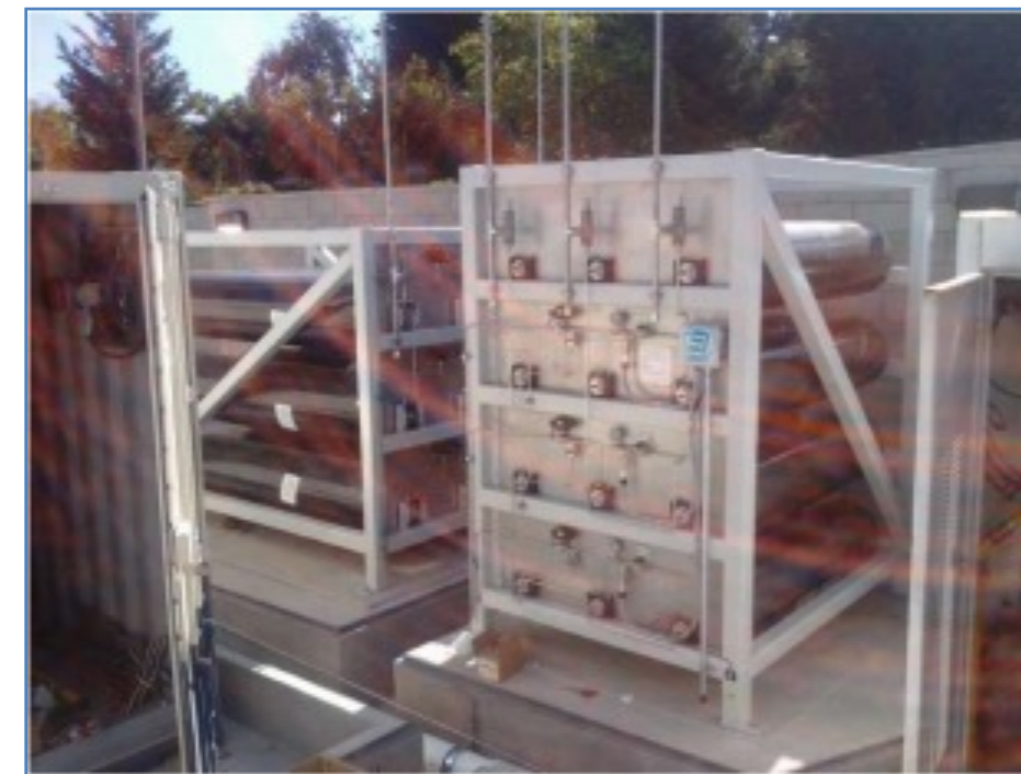
ASME steel and composite stationary storage tubes
