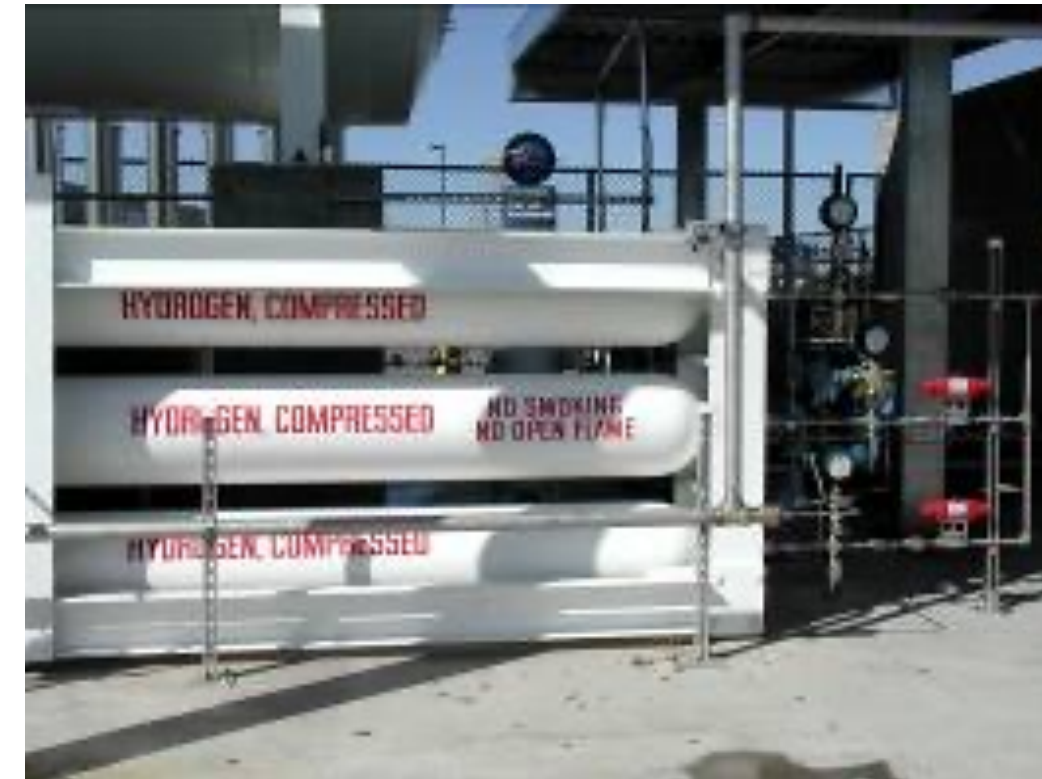
ASME steel and composite stationary storage tubes
